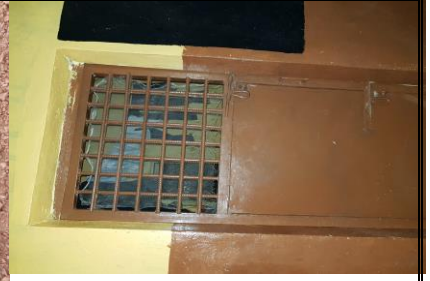
Figure 6: Completed work at the Kambia Facility
