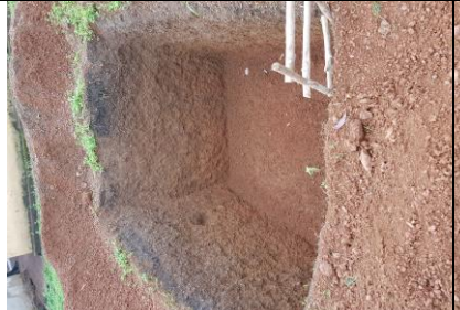
Figure 5: Work in progress at the Port Loko Facility
