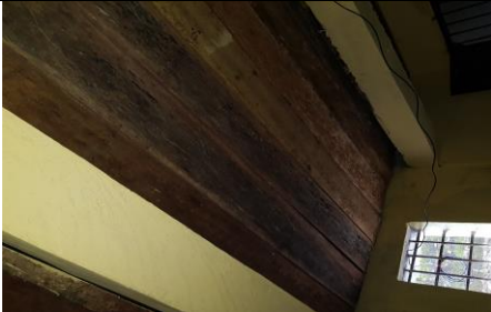
Figure 4: Completed work at the Kono Facility
