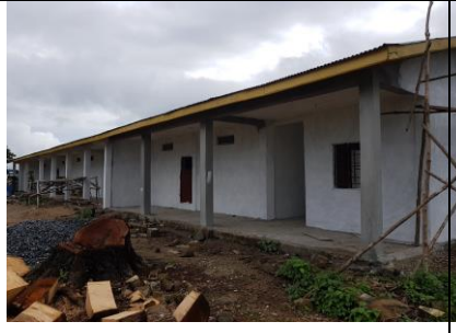
Figure 2: Work in progress at the Waterloo Facility
